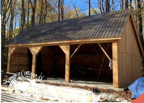
The complete pre-cut kit includes a treated sill plate and hemlock framing, pine board and batten siding, and a corrugated metal roof. Note: Pictures may reflect client upgrades and
