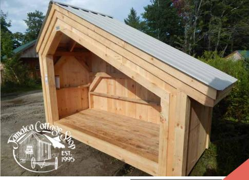
The complete pre-cut kit includes hemlock framing, pine board and batten siding, floor decking, corrugated metal roof, pine door and barn sash windows. Note: Pictures may reflect client upgrades and modifications that do not come standard.
