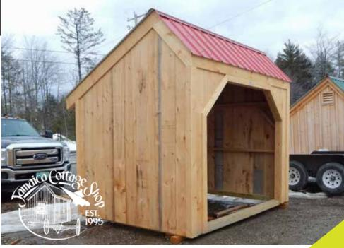
The fully assembled unit includes a treated sill plate and hemlock framing, pine board and batten siding, and a corrugated metal roof. Note: Pictures may reflect client upgrades and modifications that do not come standard.
